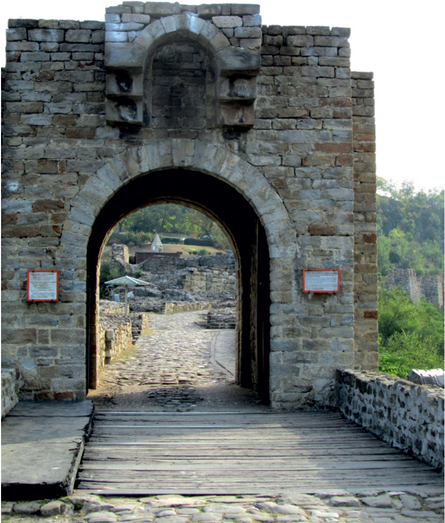
FIGURE 9 Gate 1. AUTHOR'S PHOTO.
